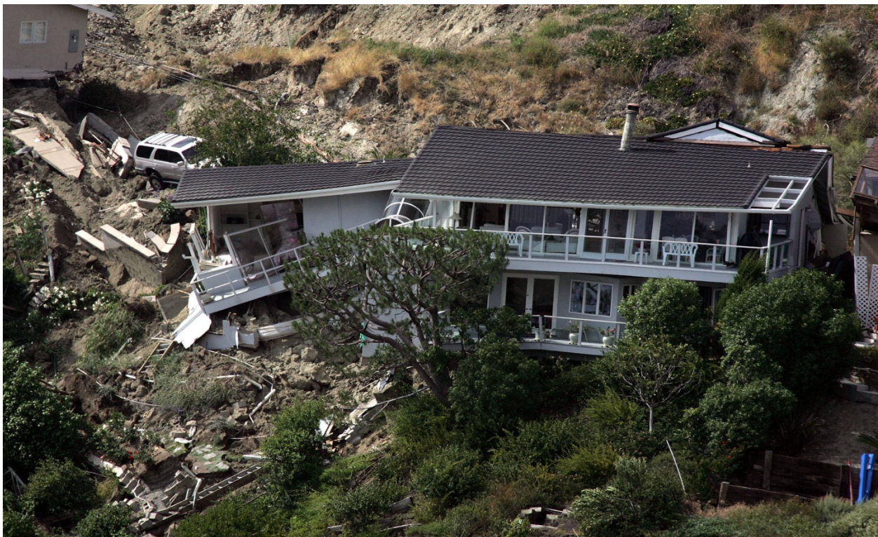
Fig 7: Landslides Destroying Homes in Southern California
