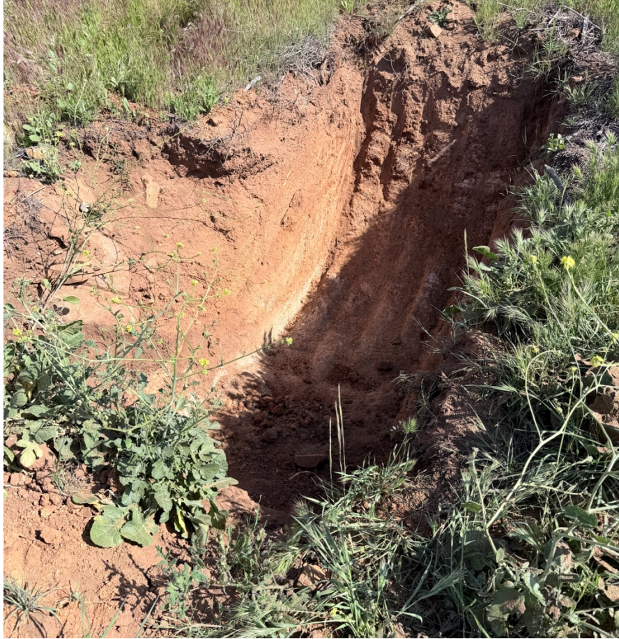
Boring 3 Depth Exceeding 5 ft
