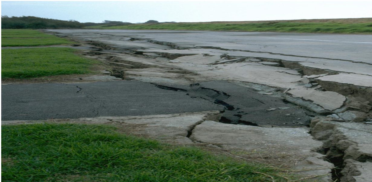
Fig 5: Lateral Spread Caused by Liquefaction
