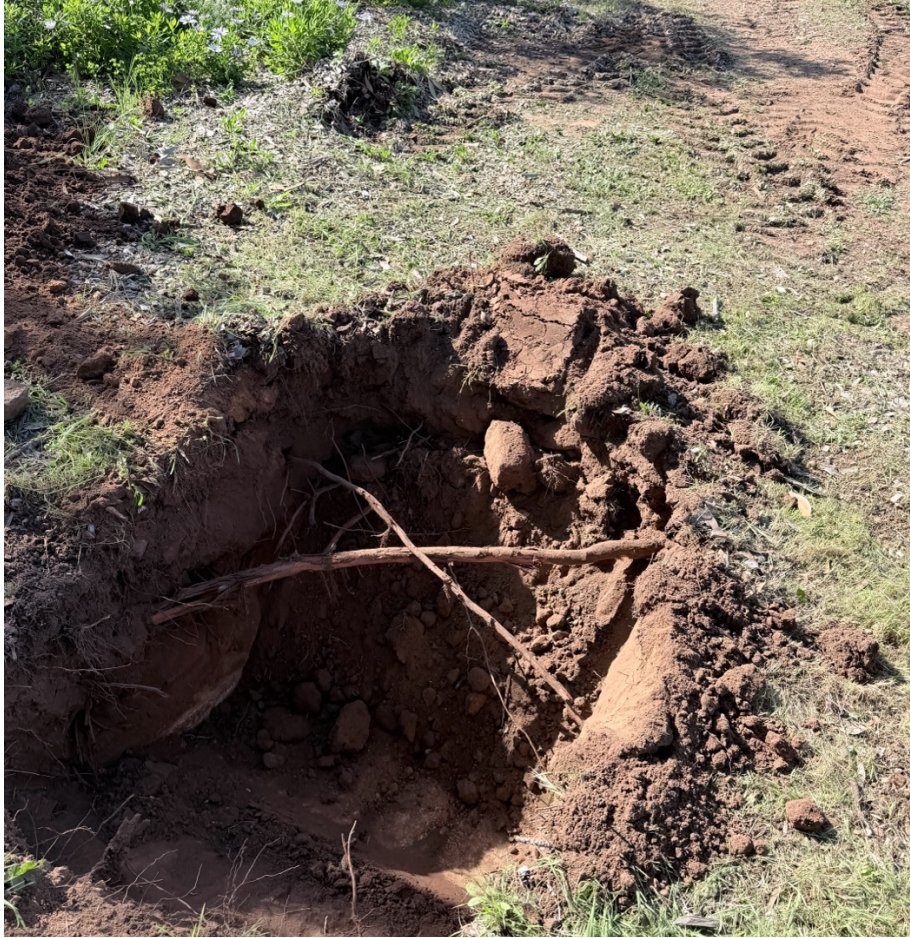
Boring 4 Depth 3 ft
